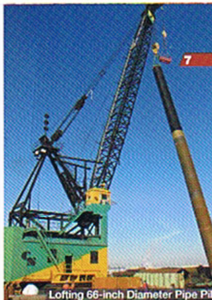
Lofting 66-inch Diameter Pipe Pile
